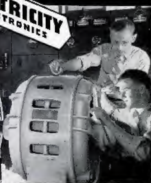
Instructor explaining operation and testing of a large Motor Generator.
